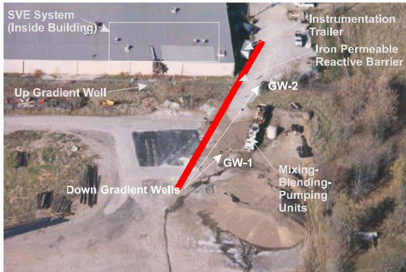
FIGURE 2. Aerial View of Site and PRB Alignment.
