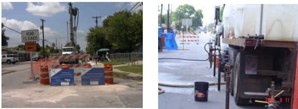
Figure 2: Photographs of PRB Installation
