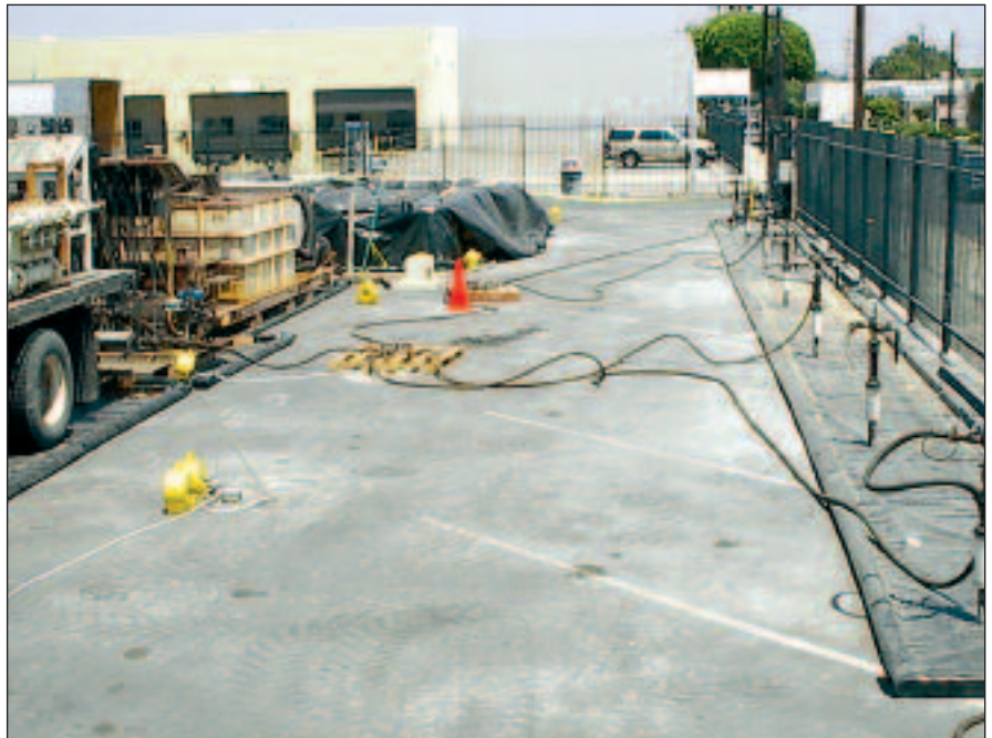
After installation, well heads will be capped and hoses removed.
