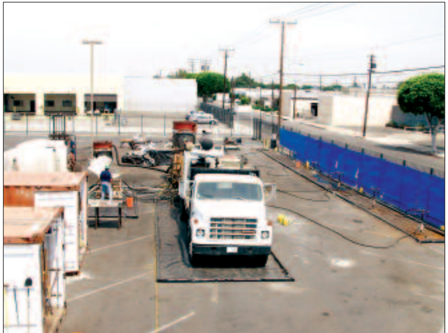
No deep trenches and large piles of soil are required.
