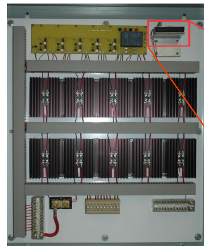
GeoSierra's Quake Defense 1/10 th MegaWatt System DC 200Volts 500Amps Seismic Switch & Controls
