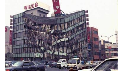
Building Destroyed by Amplified Ground Motion During an Earthquake Event
